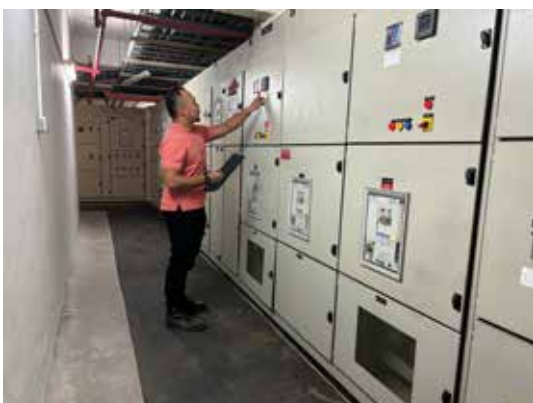
Atria Shopping Gallery's Building Management System.
