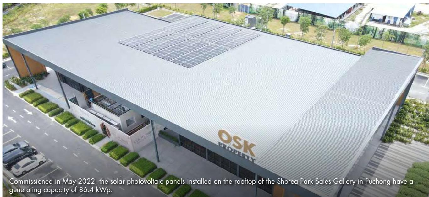
Commissioned in May 2022, the solar photovoltaic panels installed on the rooftop of the Shorea Park Sales Gallery in Puchong have a generating capacity of 86.4 kWp.
