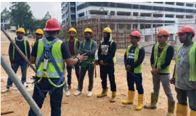
On-the-job training at a construction site.
