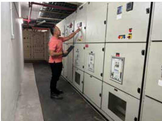
Atria Shopping Gallery's Building Management System.
